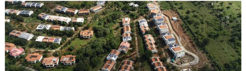
Integrated state-of-the-art rooftop solar systems for 32 row houses / villas
