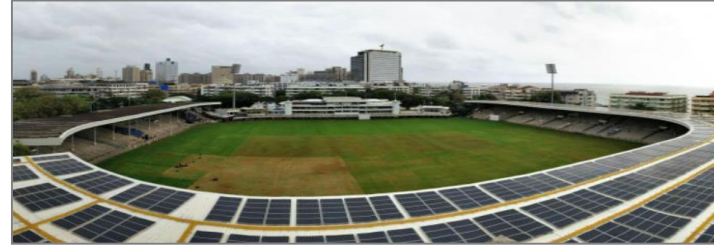
820.8 kWp at Brabourne Stadium: One of the World's Largest Solar Powered Cricket Stadiums
