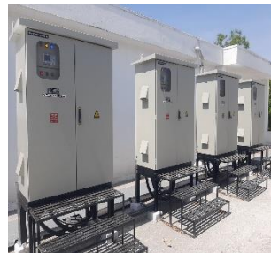
ACDB's installation with proper steps for ease of O&M
