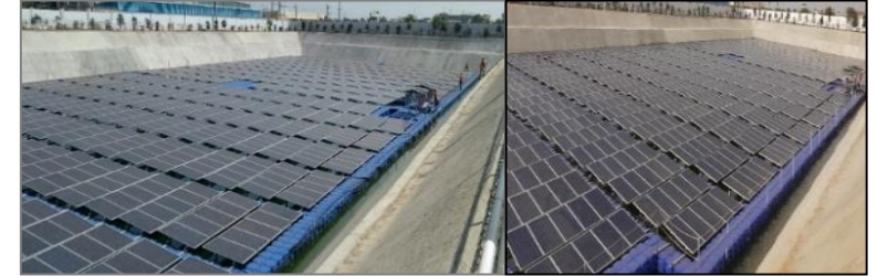
One of the first Floating Solar System built on twin ponds with a capacity of 1.4MWp at Tata Chemicals, Nellore
